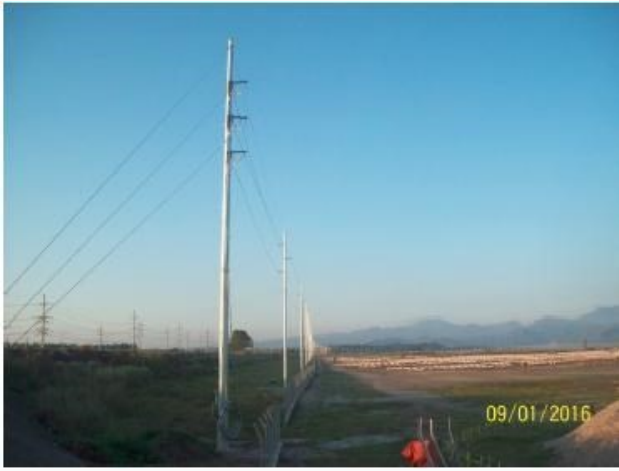
Erection of a 2km Transmission Line
